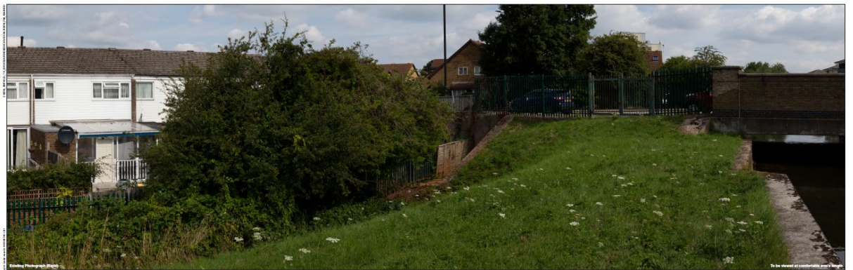
Existing Sinclair Close, looking north
